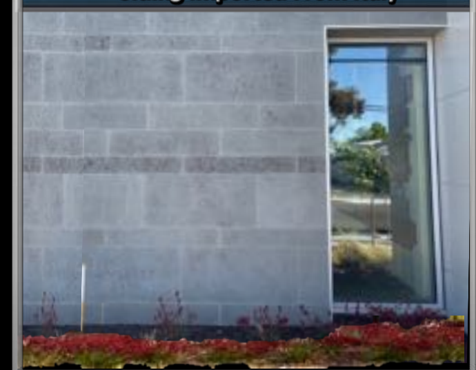
Lagos Azul Limestone Siding Imported From Italy
