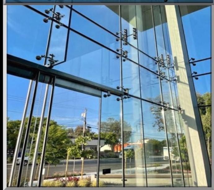
Structured Glass Lobby
